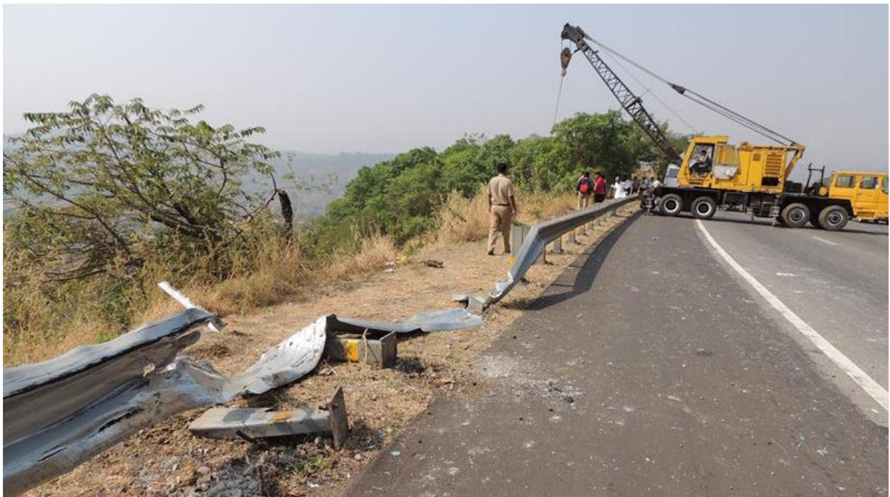
Figure 4. Cliffside barrier breached in a crash
