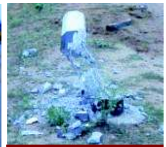
Concrete pole crushed after it was hit by a vehicle.
